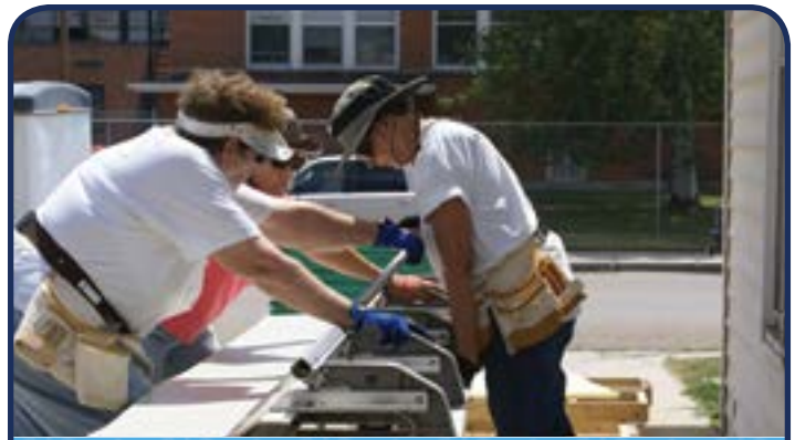
A few of the women teamed up to use the sheet metal brake to bend flashing.
