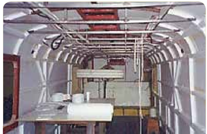
Shell with insulation
