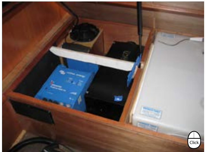
Inverter & other utilities hidden away on-board
