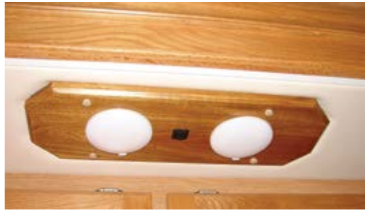
The DIY custom made LED fixture that inspired this month's LED Doctor column
