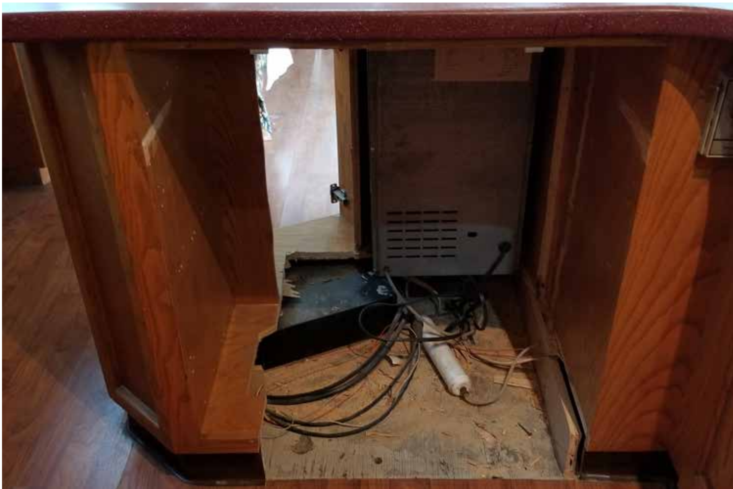
Cabinet after removing existing drawers and doors.
