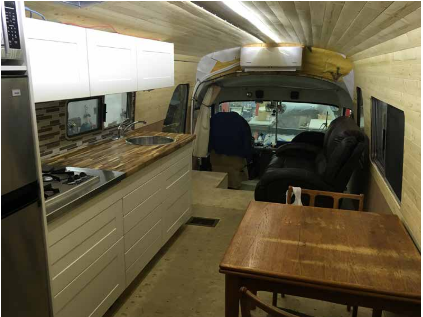
Cozy and well insulated, covered in 5/16" pine. Still some trim work to do but livable.
