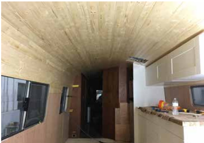
Pine covering going in, kitchen cabinets hung.
