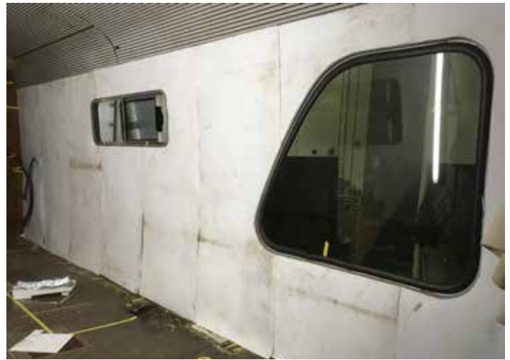
EHP held to the wall with contact cement.
