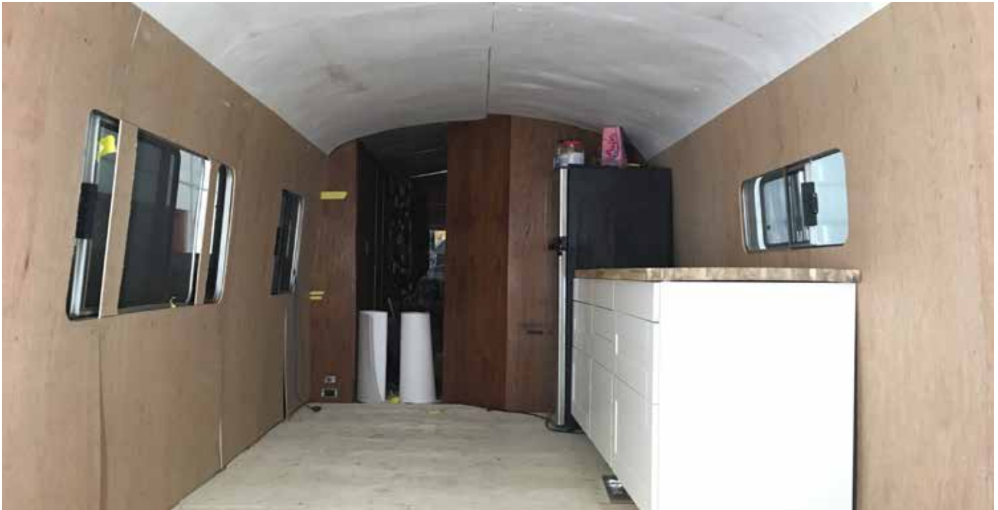
EHP can be seen on the ceiling, at only 1/8" thick it's also behind the walls and under the floor.
