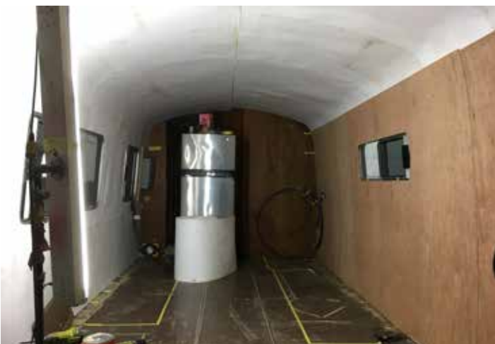
Walls and ceiling complete, new luan on the wall.
