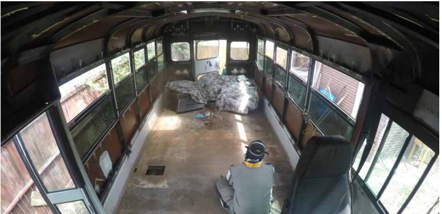
Cleaning the Rust Off of the Floors.
