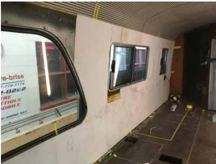
EHP starting to go up on curb side wall.
