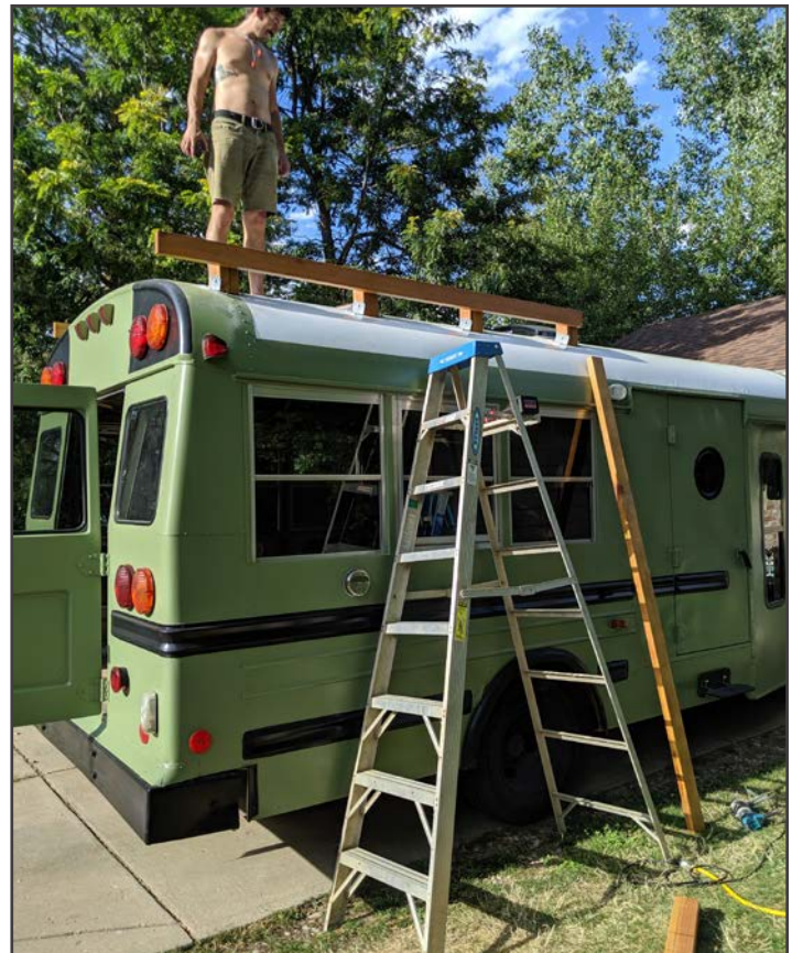
Building the Roof Deck.
