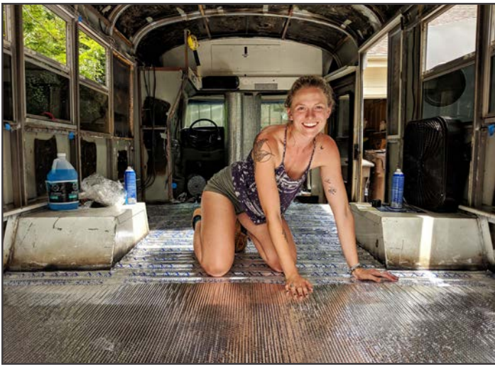
Adding the floor insulation. While Reflectix doesn't do too much, we couldn't spare any space. AJ's head scrapes the ceiling even with such thin insulation.
