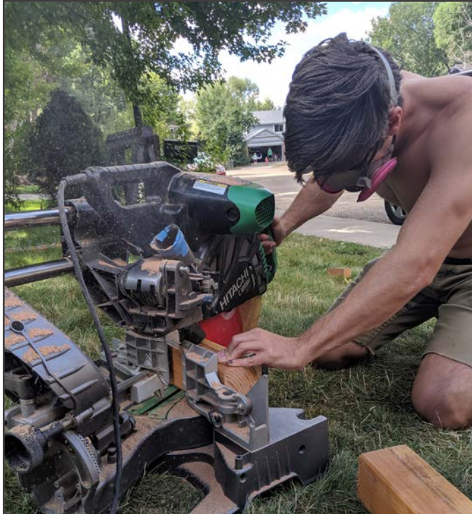
Cutting wood for the roof deck.
