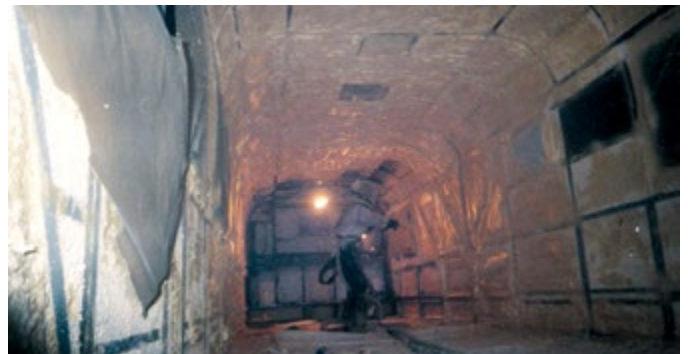
We chose spray foam insulation.
