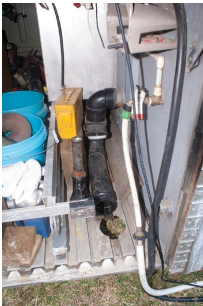
Waste water dump, fresh water connection , & 50A shorepower cord.
