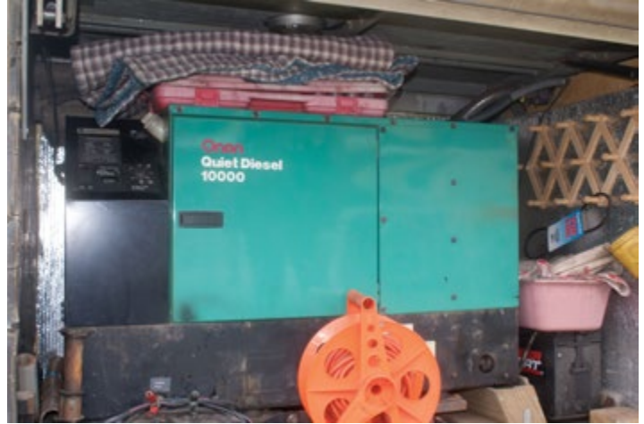
10KW diesel generator
